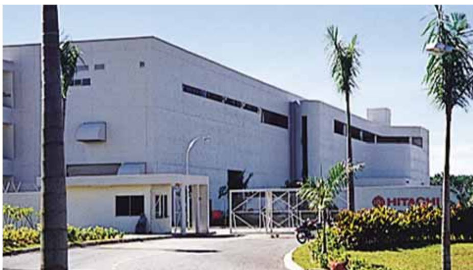
Hitachi Air Conditioning Products (M) - HAPM Proizvodni pogon - Kuala Lumpur, Malaysia
